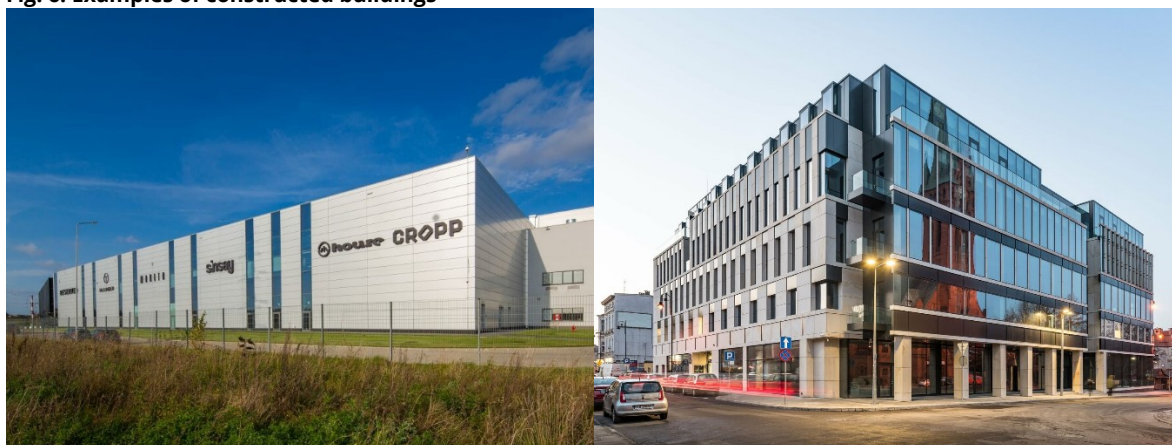
Fig. 6. Examples of constructed buildings
