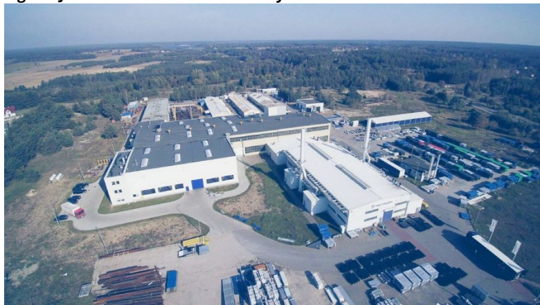
Fig. 2. PJP Makrum: Production facility
