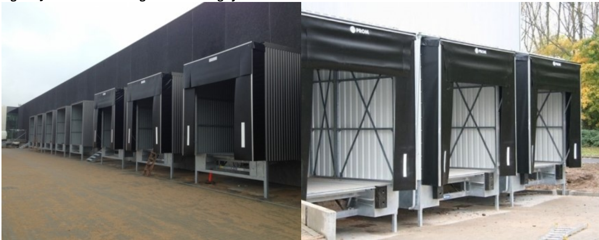
Fig. 1. PJP Makrum: Loading and unloading systems
